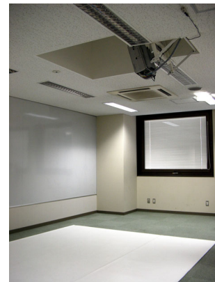
Fig. 3: Complete view of the system
